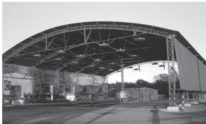
Figure 1. The holding area with environment control at the slaughterhouse.
